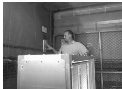
The M-Series air handler - with its modular components, bolted construction, and removable panels - readily lends itself to the special needs of the renovation, retrofit, and replacement markets. To integrate new features, simply separate the existing modules and add, enhance, or replace components.
