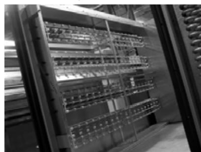
Figure 65. Energy wheel module
