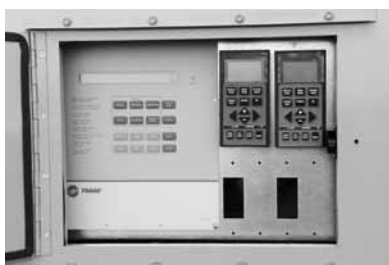
Figure 13. Human Interface Panel (HI)
